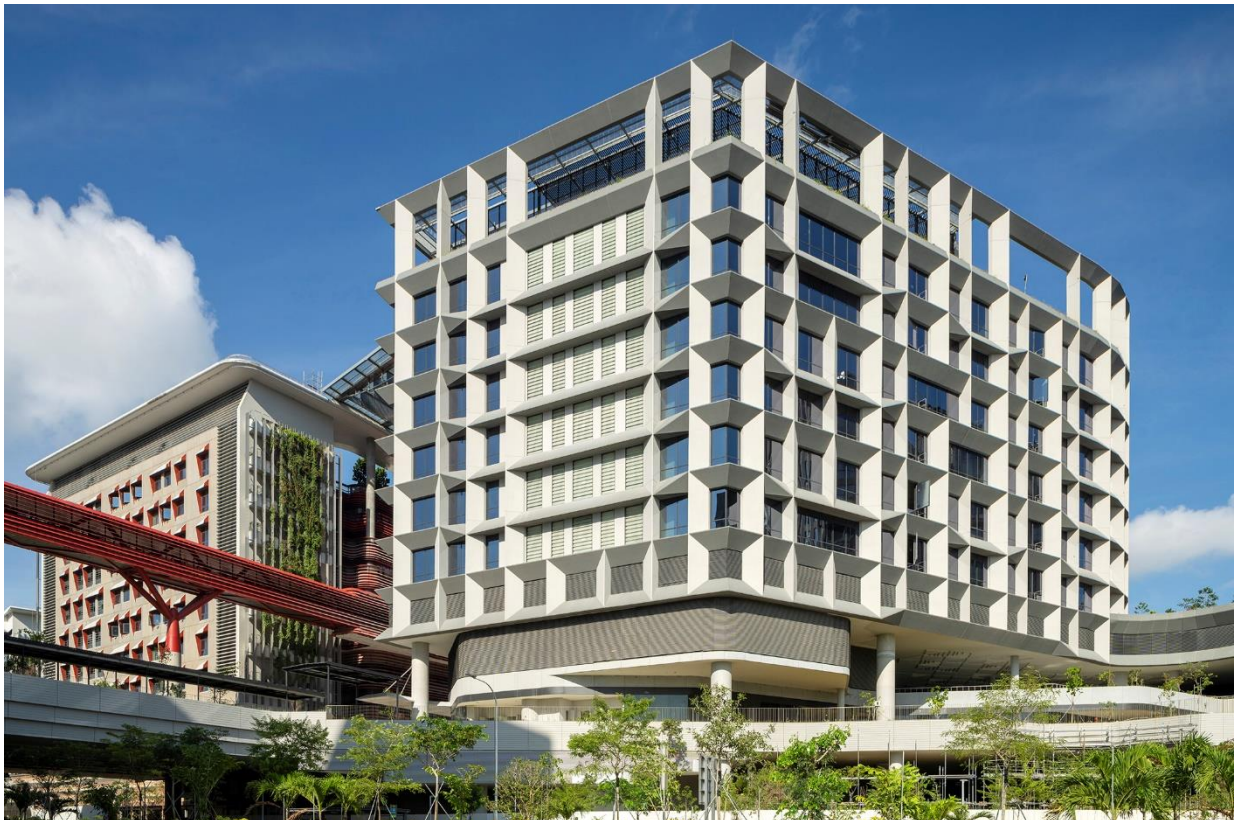
Punggol Digital District (Credit: Darren Soh for JTC)
